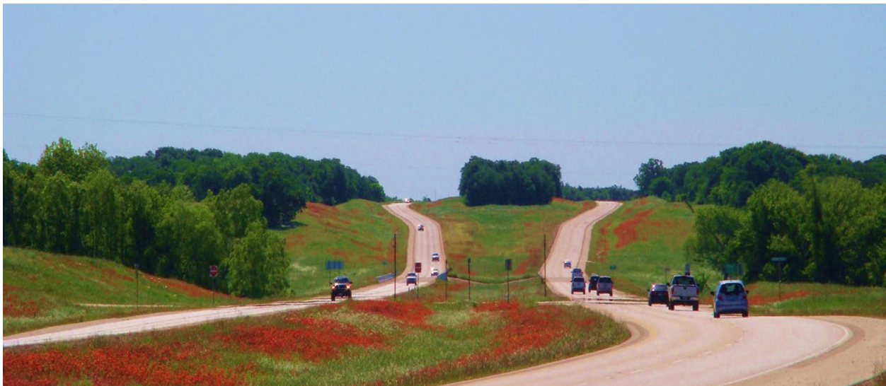
Figure 5. State Highway 47 in Bryan, TX (Courtesy TTI).
